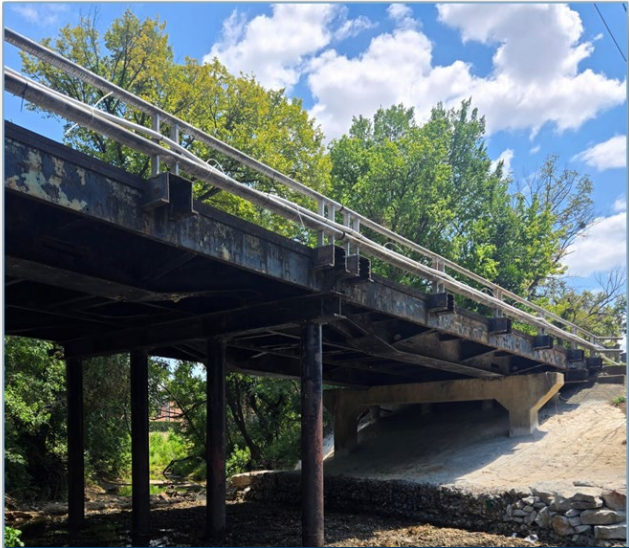
Heritage Avenue Bridge
