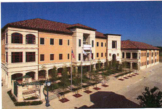
Colleyville City Hall
